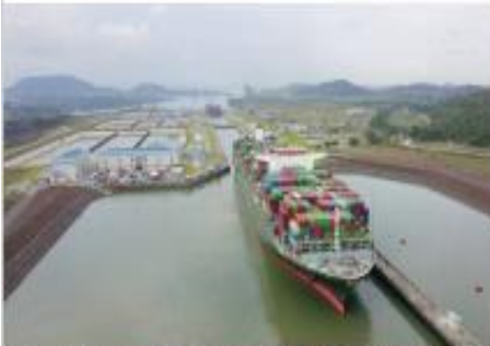
above: The neo-panamax locks of the Panama Canal accept 20 rows-wide container vessels with a length of up to 370.3 meters. Draft is temporarily restricted from 50 to 44 feet.
